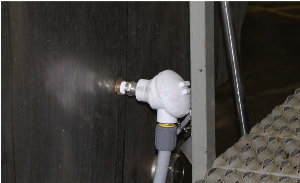
After a brief discussion and a quick look at the location, it was decided that a Burns Series 300L spring loaded RTD for use in the existing thermowell would provide the accuracy and durability Jason required. The addition of a polypropylene connection head
